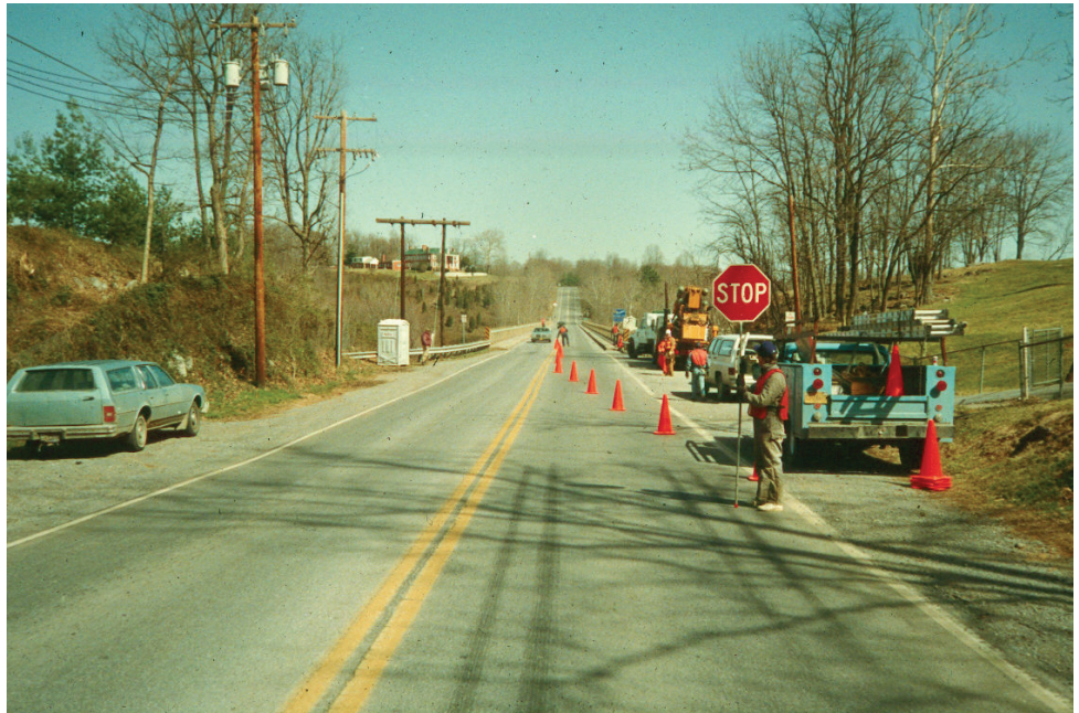
Figure 3.1.4 Traffic Control Operation
