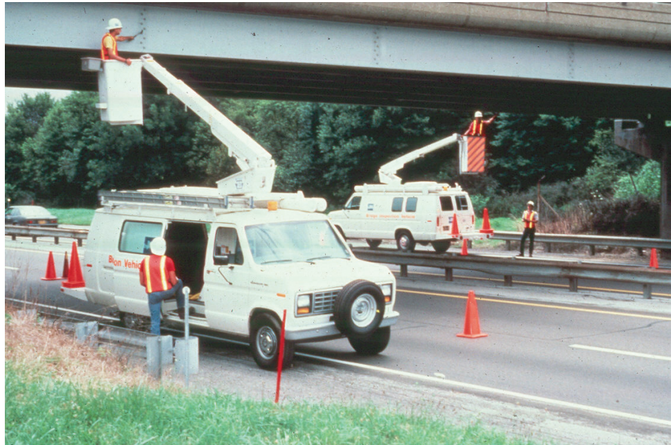
Figure 3.3.3 Inspection Vehicles with Flashing Light
