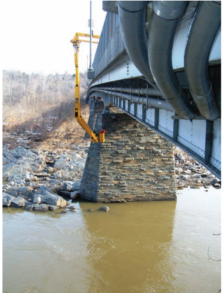
Figure 3.5.16 Underbridge Inspection Vehicle
