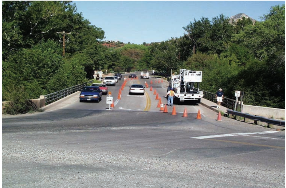
Figure 3.3.1 Traffic Control Operation
