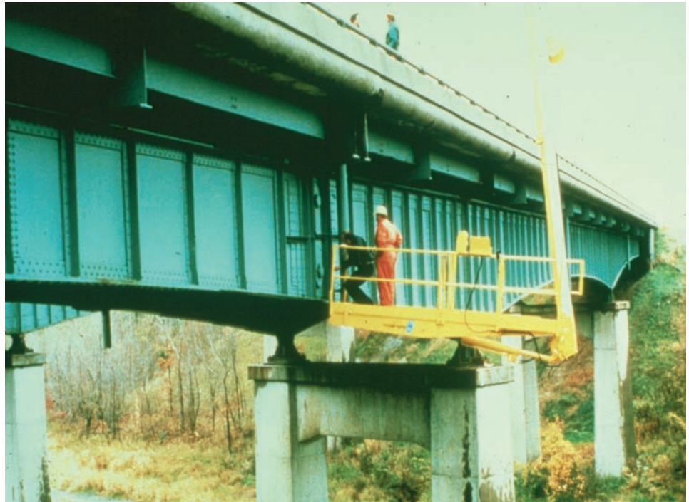
Figure 3.5.17 Underbridge Inspection Vehicle (Snooper) with Platform
