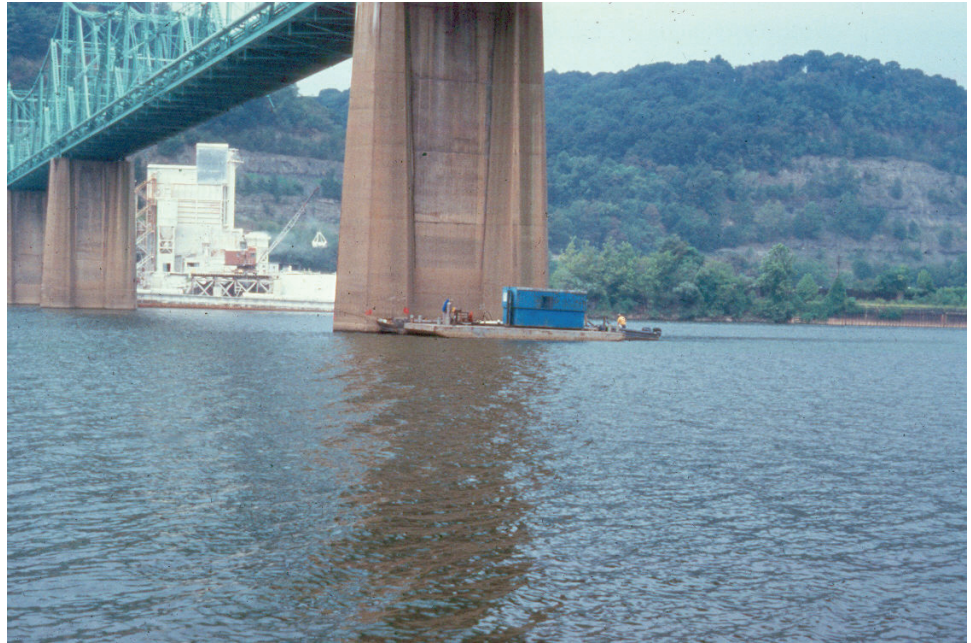
Figure 3.5.6 Inspection Operations from a Barge
