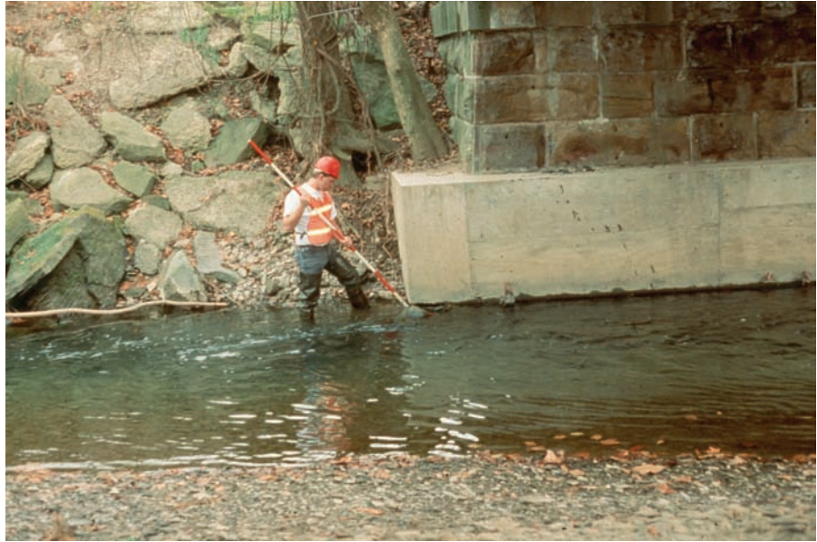
Figure 3.1.5 Inspection for Scour and Undermining
