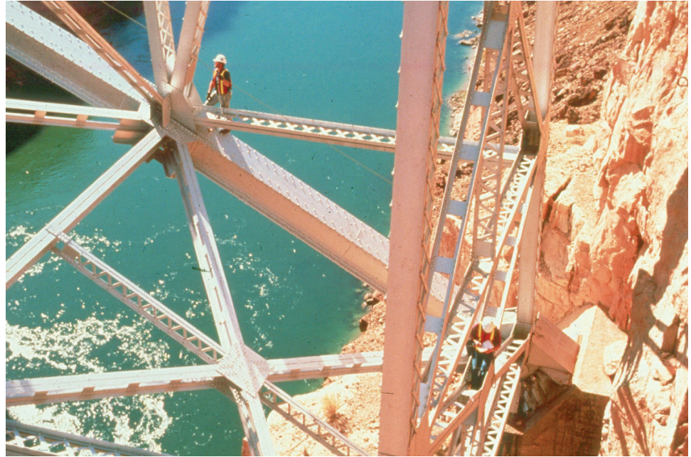
Figure 3.2.7 Inspection Involving Extensive Climbing
