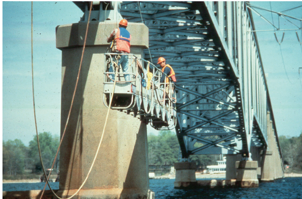
Figure 3.5.3 Rigging for Substructure Inspection
